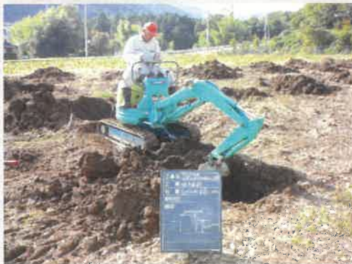
植穴掘削 W1,000mm × D600mm
